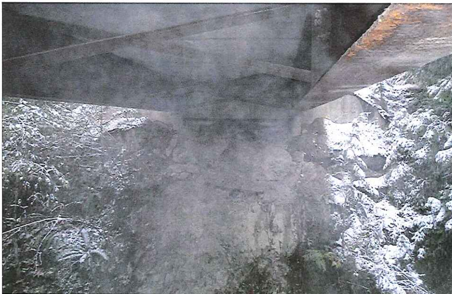
CK2132 Abutment Left Bank
