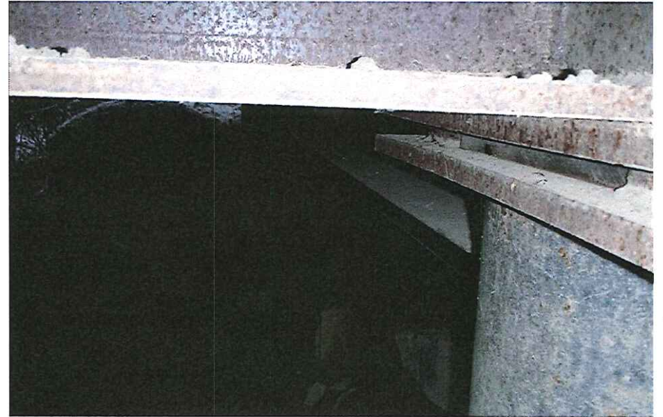
CK2132 Abutment Left Bank #2
