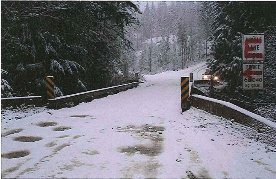
CK2132 Approach Right Bank
